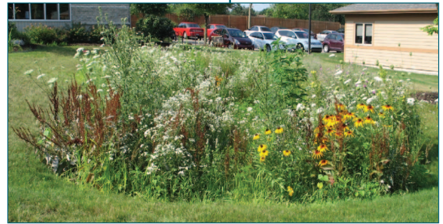
Figure 1. Rain garden built to capture rainwater from a parking lot and roof.
