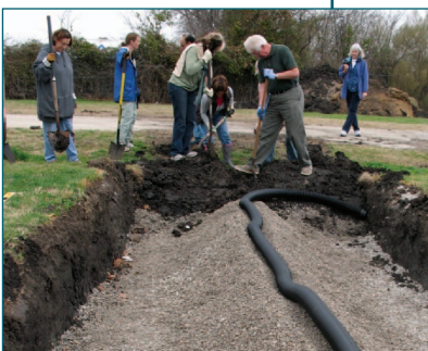
Figure 5. Placing a perforated pipe on top of the gravel.
