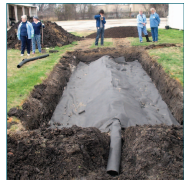
Figure 6. Placing the filter fabric.
