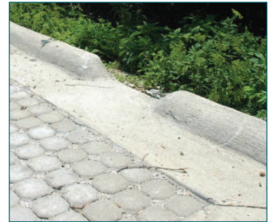
Figure 4. Curb cut opening. (Source: USDA, NRCS)
