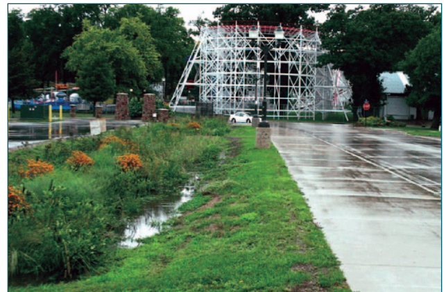
Figure 2. Rain garden built as an island in a parking lot. (Source: United States Department of Agriculture, Natural Resources Conservation Service)
